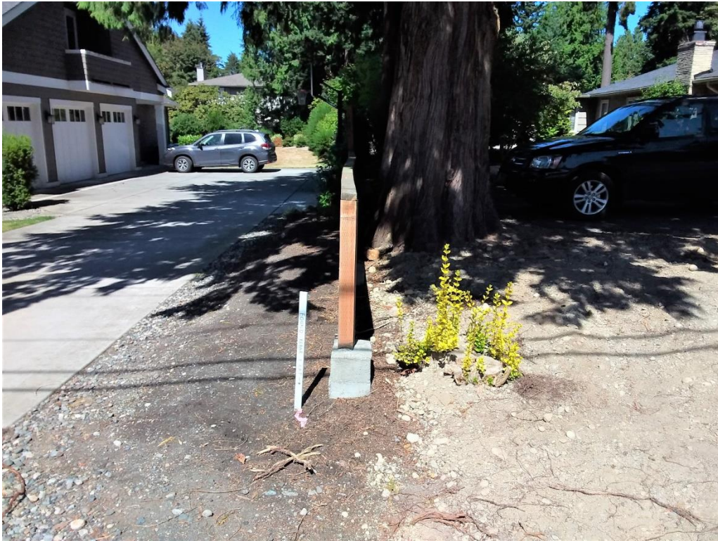
Figure 9. Photo taken during the August 2020 site visit looking north up the west fence line at the base of the #1 cedar. Note proximity of neighbor's driveway.
